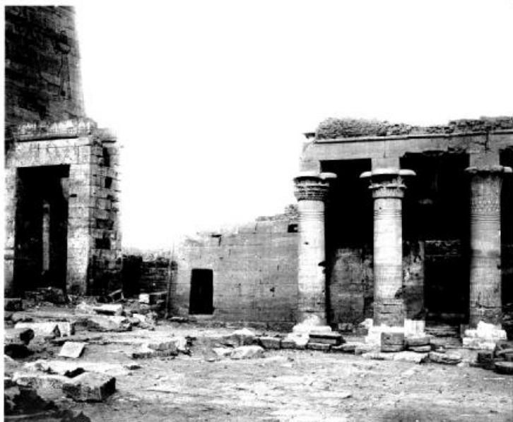
East Colonnade (VI) Columns 13 to 17.
